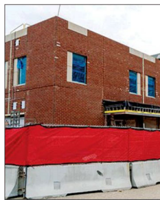
An addition to Northern Light's Mercy Hospital is under construction on Monday. Personnel are working on the site.
